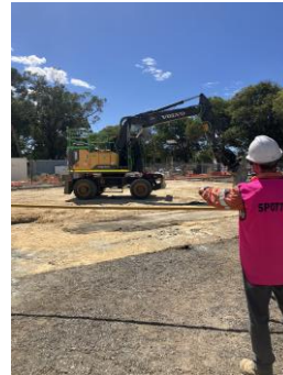
Image 1 – Providing guidance to operators of heavy machinery.
