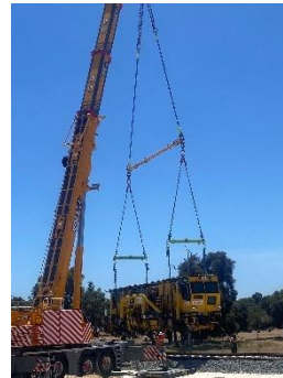
Photo 5 – Use of Crane.
