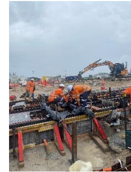
Photo 2 –Manoeuvring parts onsite.
