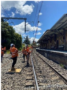
Photo 4 – Use of equipment for testing electrical currents.
