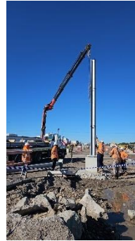
Image 2 – Installing masts.
