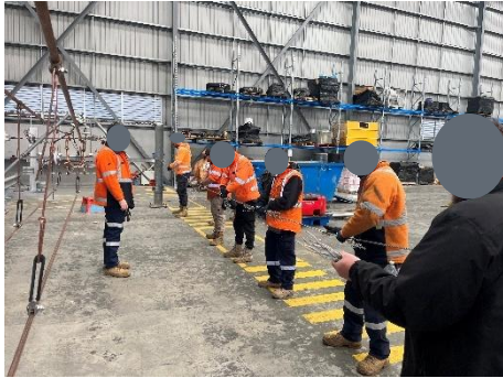
Photo 1 – Building/assembling parts on the ground.
