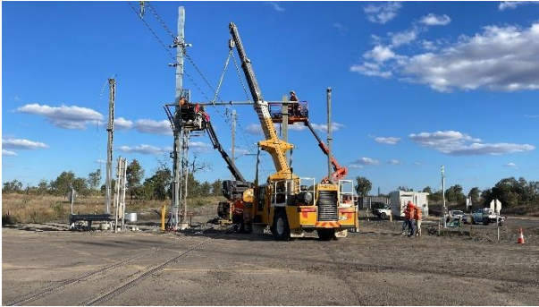
Image 1 – Installing masts overhead.
