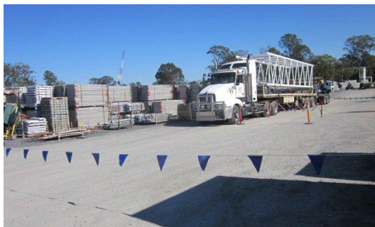
IMAGE 1 - Examples of means of setting up a quick effective LUEZ demarcated in a manner which is fit for purpose for the nature of the loading/unloading environment
