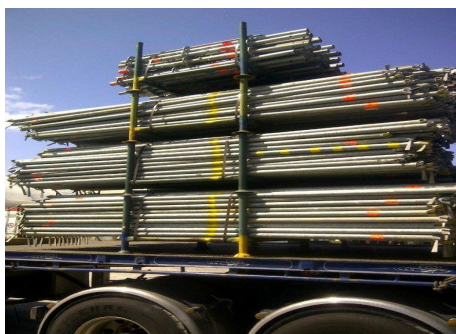
IMAGE 3 - Poor practice – no safe access for the Dogman
