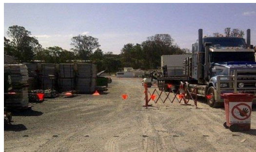
IMAGE 1 - Examples of means of setting up a quick effective LUEZ demarcated in a manner which is fit for purpose for the nature of the loading/unloading environment
