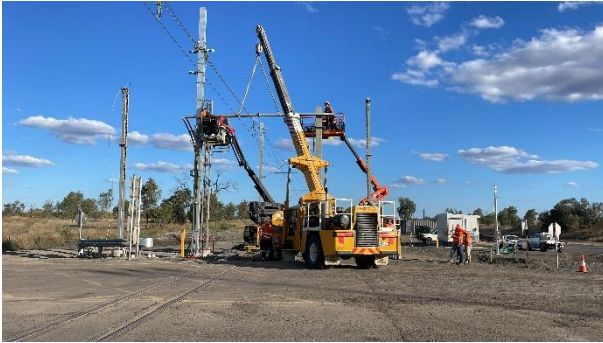
Image 1 – Installing masts overhead.
