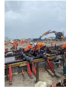
Photo 2 –Manoeuvring parts onsite.
