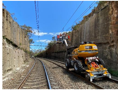
Photo 2 – Operating Cherry Picker at Height.
