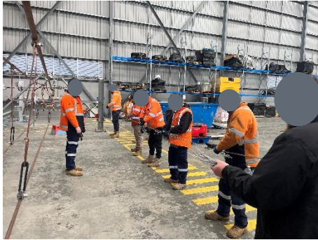
Photo 1 – Building/assembling parts on the ground.
