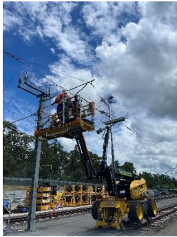
Photo 1 – Operating Cherry Picker at Height.
