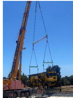
Photo 5 – Use of Crane.
