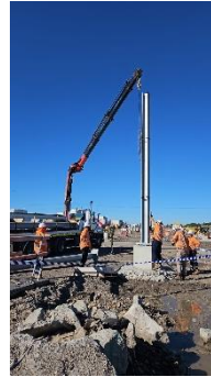
Image 2 – Installing masts.
