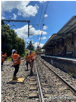
Photo 4 – Use of equipment for testing electrical currents.
