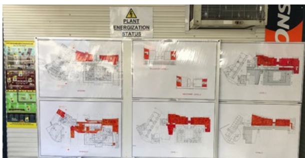
Figure 7 Example of energisation status noticeboard
