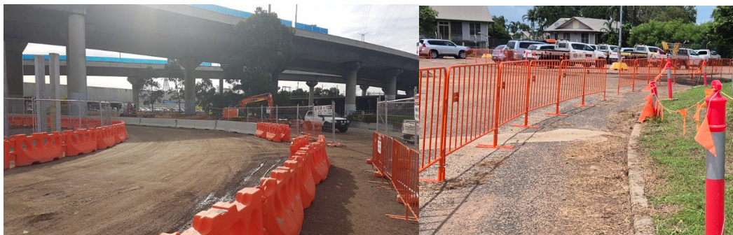
Example of Physically Separated Pedestrian from operating vehicles.
