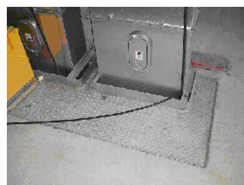
Figure 9 From Underside: Metal Flooring with holes for future services. Note ply protection.
