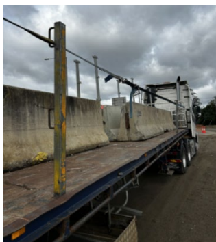
Example of a poor webbing type edge protection system
