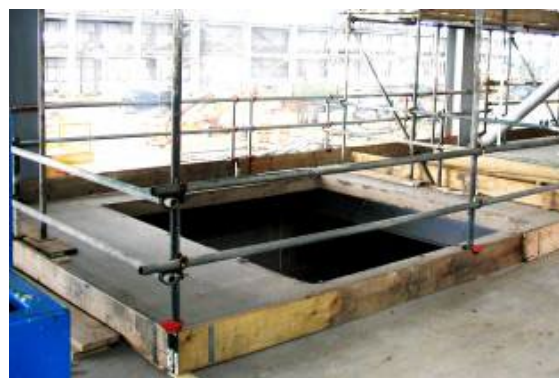
Figure 5 Example of protection to large penetration
