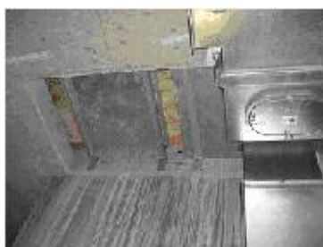
Figure 8 Metal Riser Flooring with 65mm perimeter upstand
