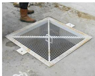
Figure 7 Example of temporary cover awaiting fixing to slab
